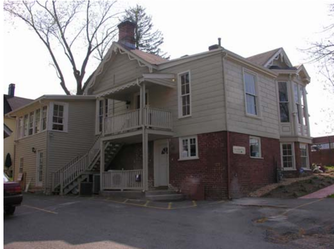
Built in 1860 ~ on the National Historic Register
